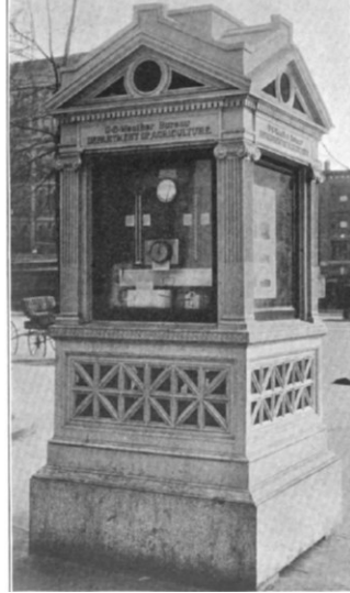
Figure 24. A Weather Bureau Kiosk in Washington, DC, providing a public display of real-time instrument recordings (Source: MWR 1909:90).
